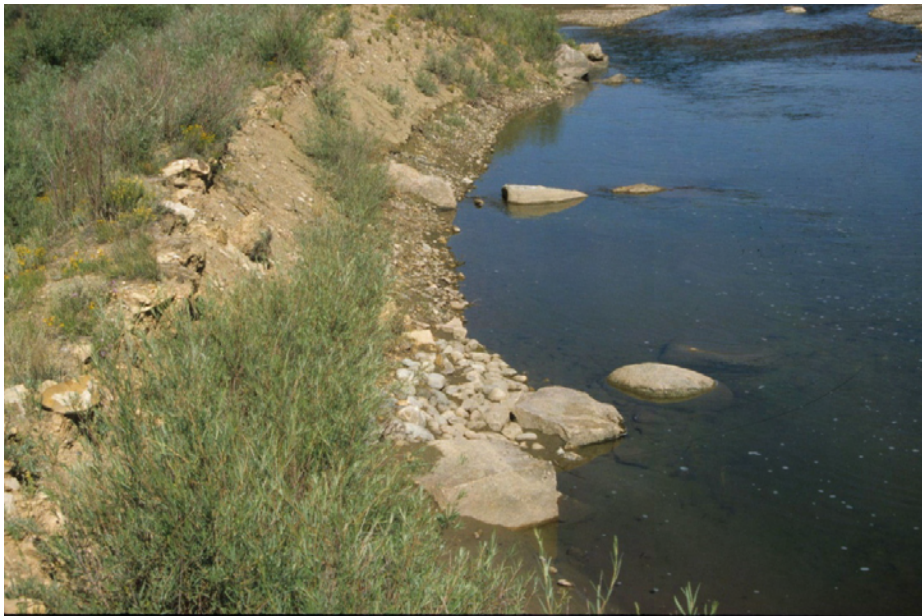
Figure A.15. Half cross (boulder) vane.
