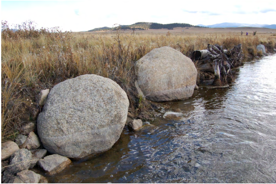
Figure A.18. Single boulder deflector.
