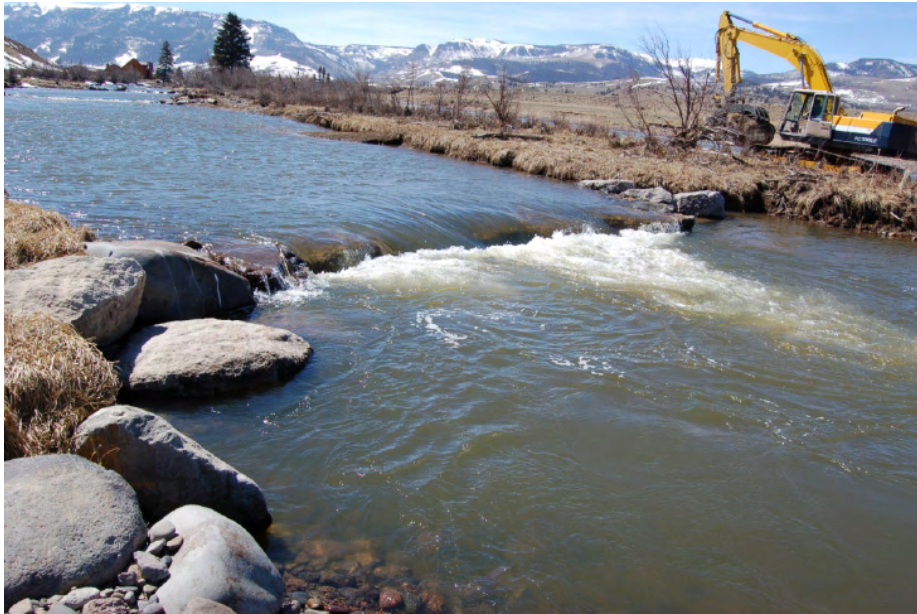
Figure A.14. Cross vane.
