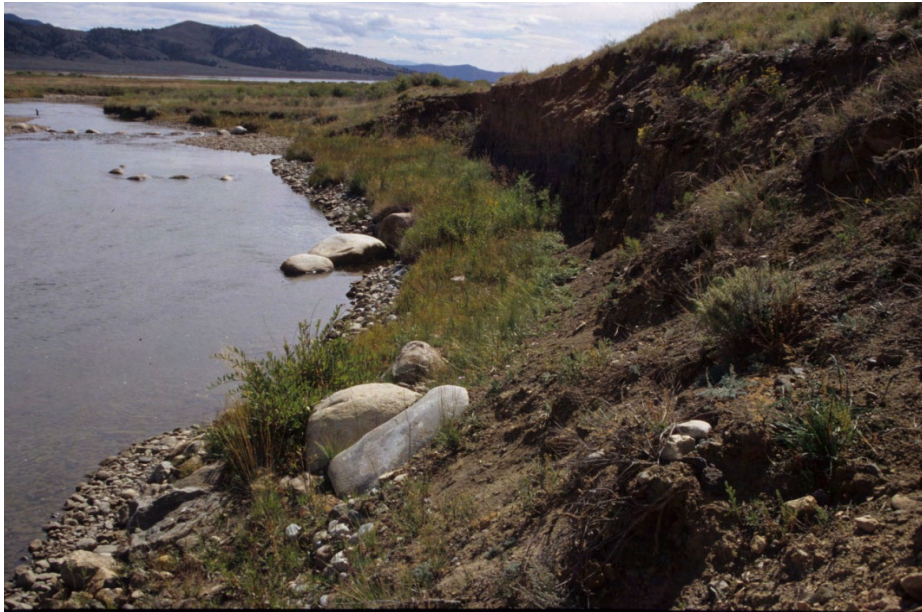
Figure A.8. Add a riparian bench with a cobble toe.
