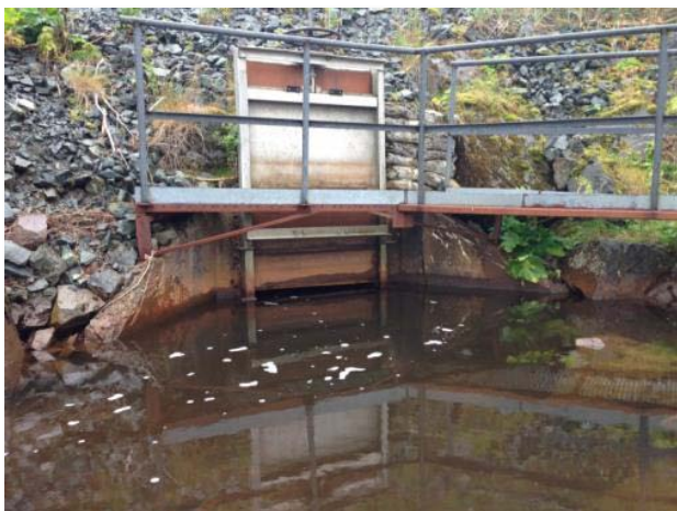
Figure 8: Spill control gate on Culvert #5 (lower and upper) 2014.
