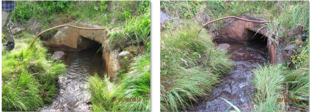
Figure 4: Culvert #3 after trash rack removal 2013 (L); 2014 (R).
