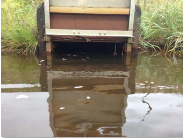
Figure 7: Spill control gate on Culvert #3 and new reference mark 2014.
