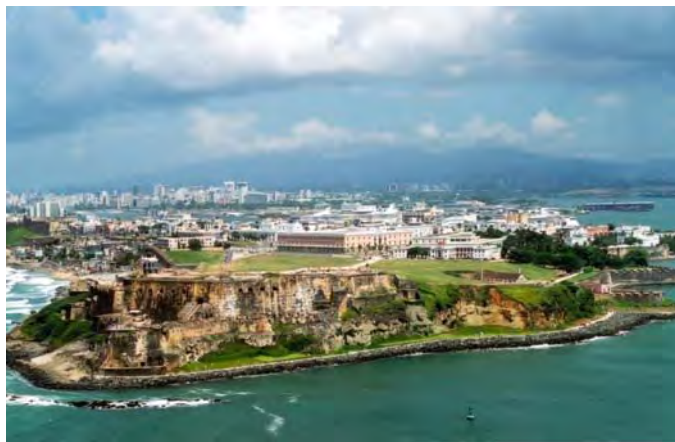
Figure 4-2. Oblique Aerial View of Old San Juan
