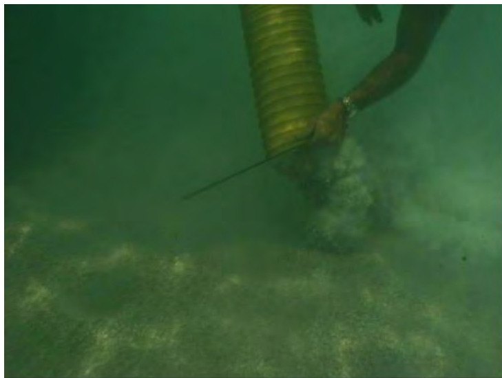
Figure 2-3. Fill Being Deposited in a Blowhole using a Large-Diameter Flexible Hose
