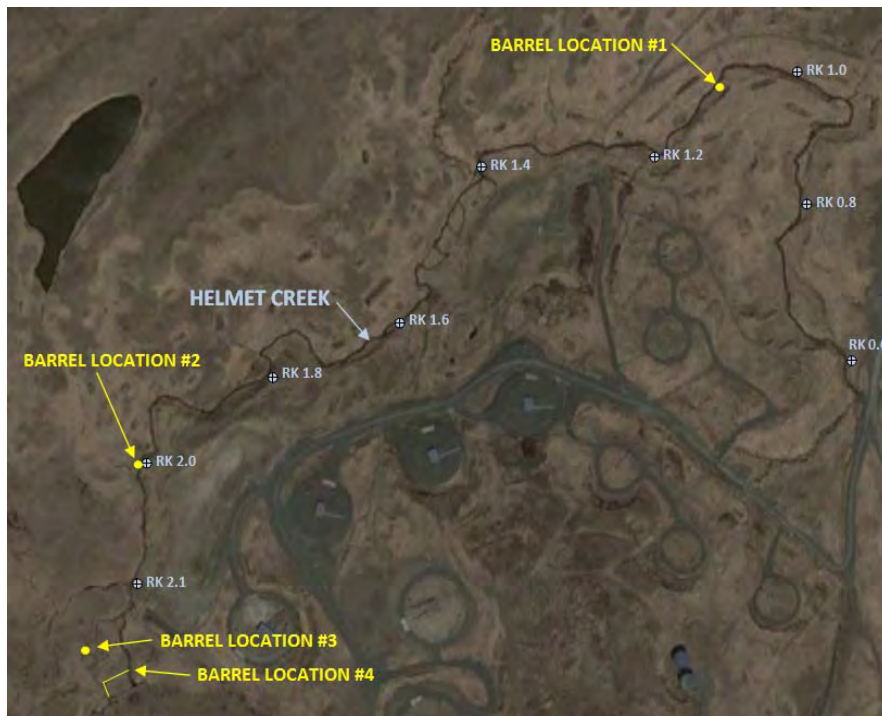
Figure 2: Upper Helmet Creek showing structures
