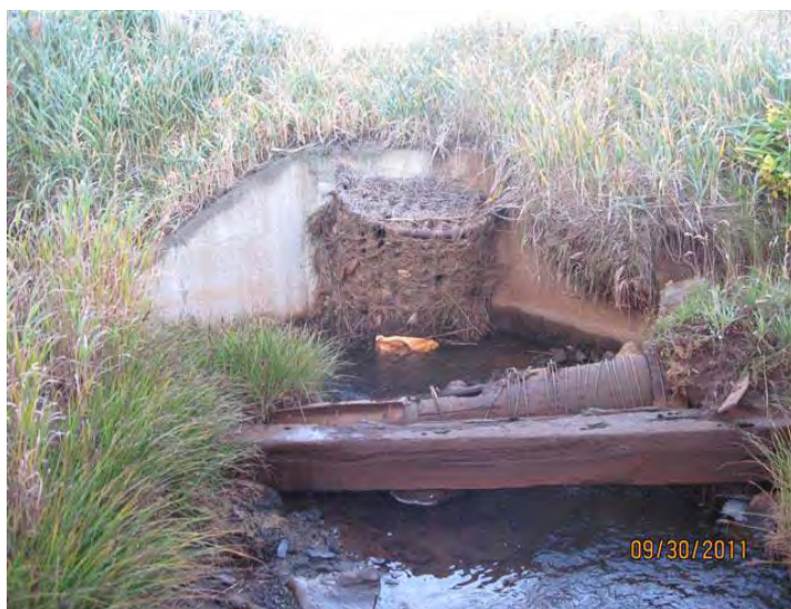
Figure 3: Wood stave pipe and timber
