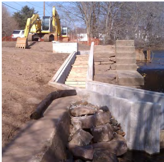
Figure 3. Construction of fishway at Wallace Dam in Wallingford. Photo by Steve Gephard.
