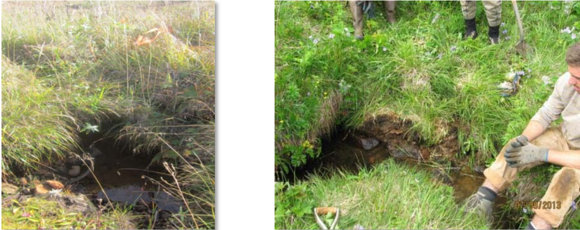
Figure 15: Culvert complex (Site #4) before and after plugging
