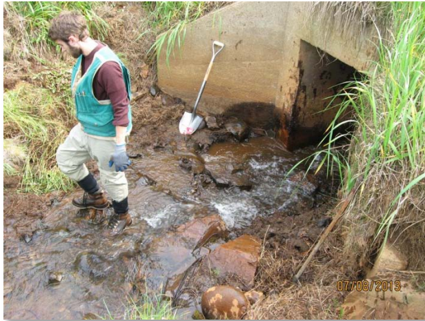
Figure 5: New channel bed created at Culvert #2
