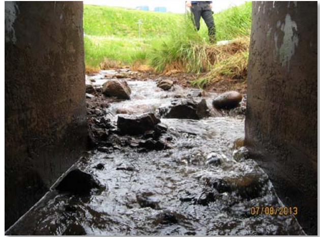
Figure 5: New channel bed created at Culvert #2
