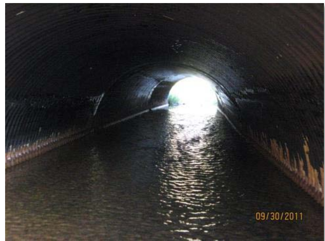
Figure 9: Fish passage conditions in Culverts #3 and #4
