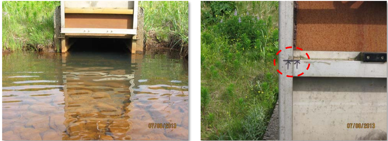
Figure 7: Spill control gate on Culvert #3 and reference mark (highlighted)
