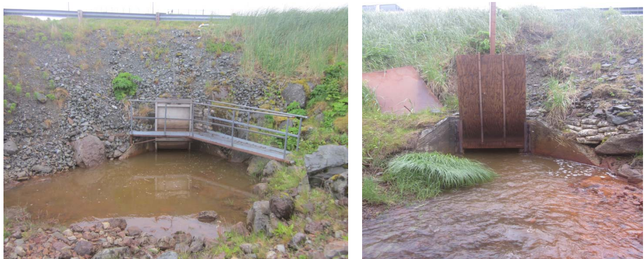
Figure 8: Spill control gates on Culvert #5 (lower and upper)
