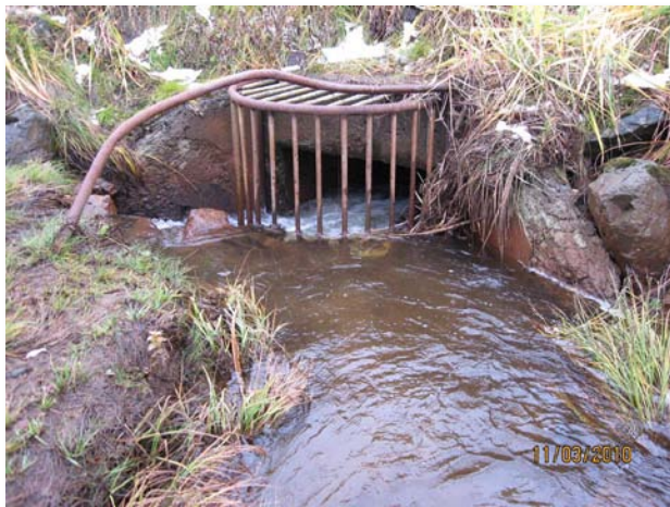
Figure 6: Culvert #3 before (Left - 2010) and after (Right - 2013) trash rack removal
