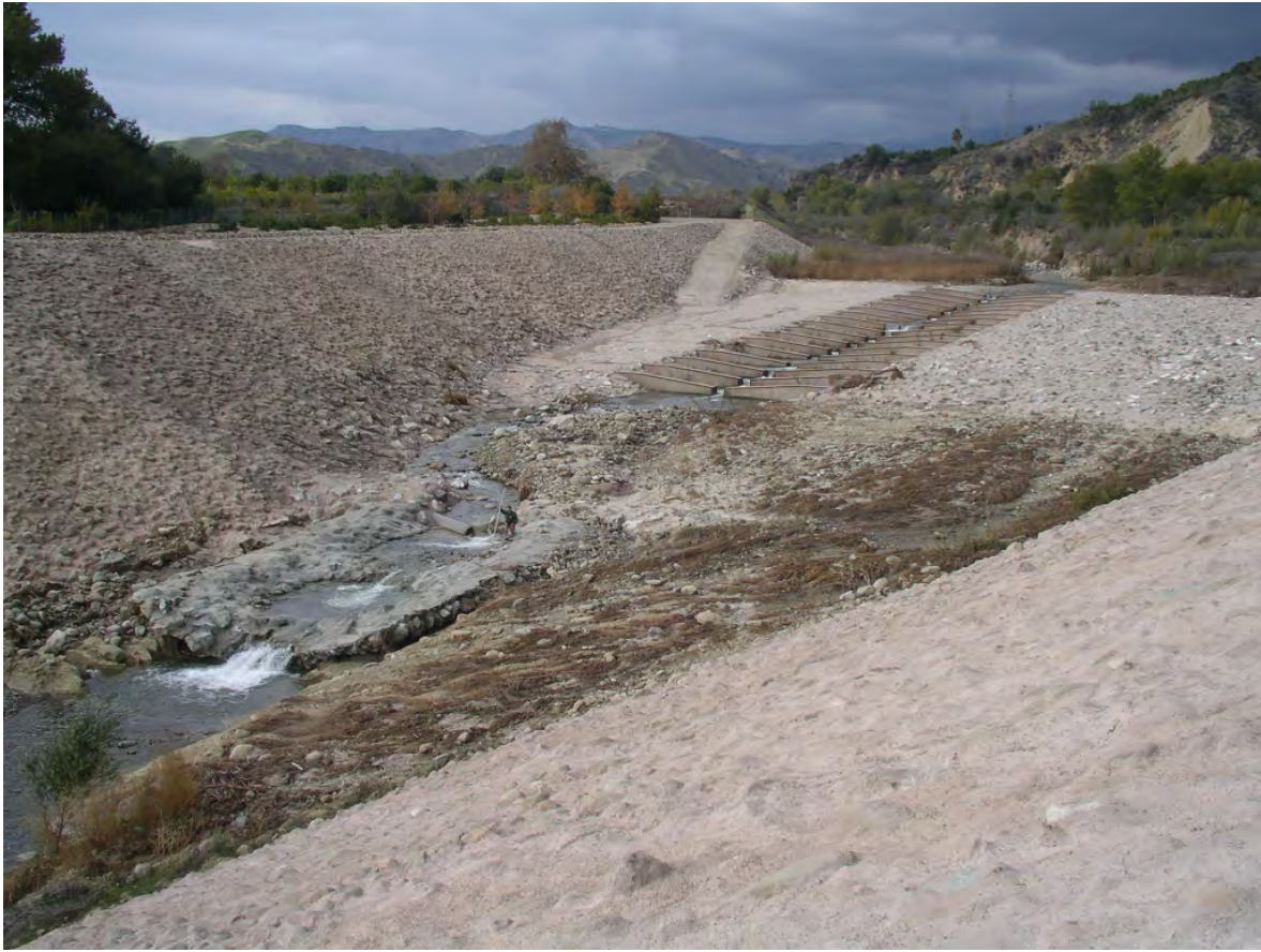
Grade control and fishway before 2005 failure
