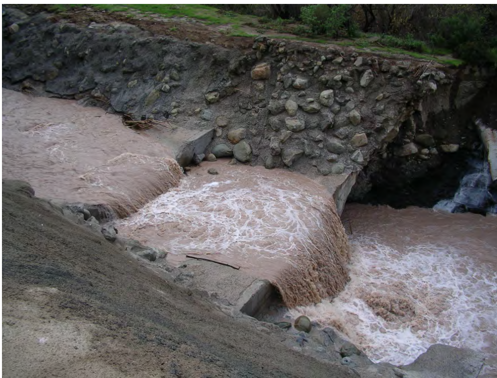
Failure of downstream grade controls following 2005 flood
