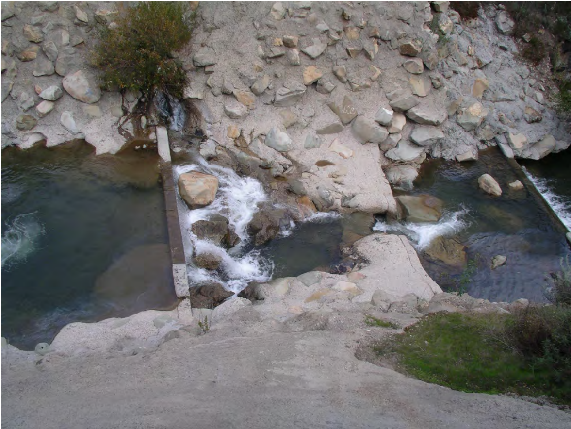
Downstream grade controls before 2005 flood
