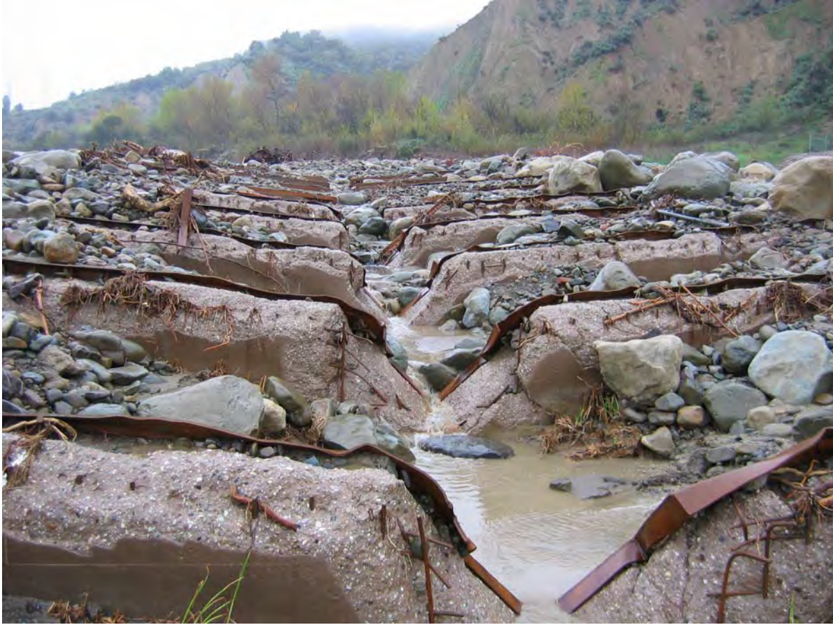
Fishway failure following January 2005 flows
