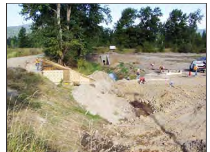
East field water control structure construction, September, 2007.
