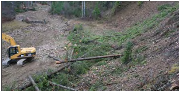
Constructing slope protection along Trapper Creek, 2007.
