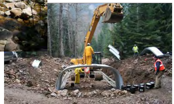
Installing replacement culvert at Langlois Creek, November 2007.
