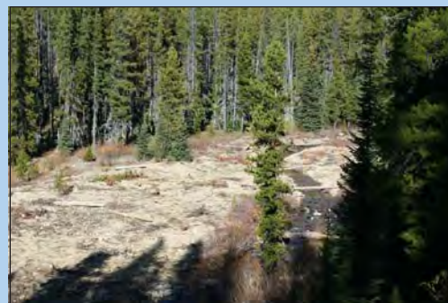
(10/29/08) Upstream end of project area - stream construction area begins.
