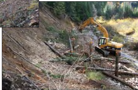
Constructing toe slope protection with onsite materials, near Calusa Creek, August, 2007.
