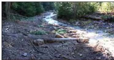
Highland Creek floodplain stabilization, October, 2008.
