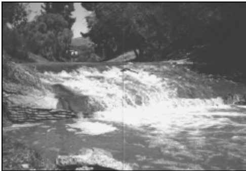
Figure 12. Photograph of Prefumo Creek, Fish Barrier PR-1-3B.
