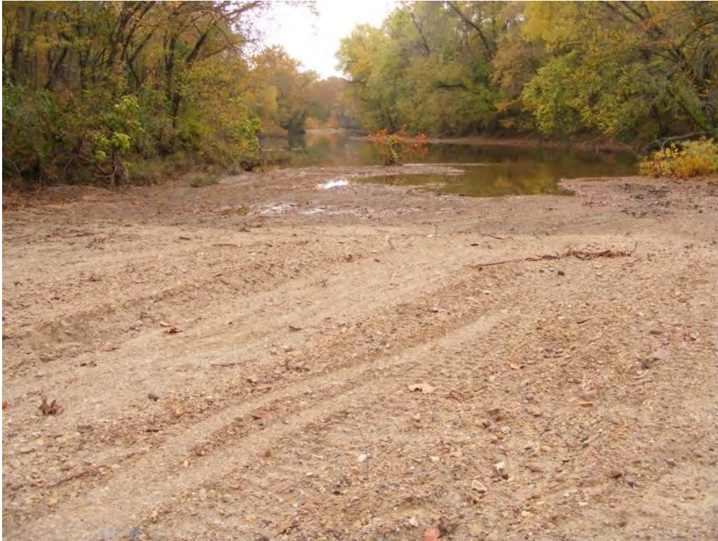
Looking upstream across excavated bar head. Notice excavator tracks and flat topography.
