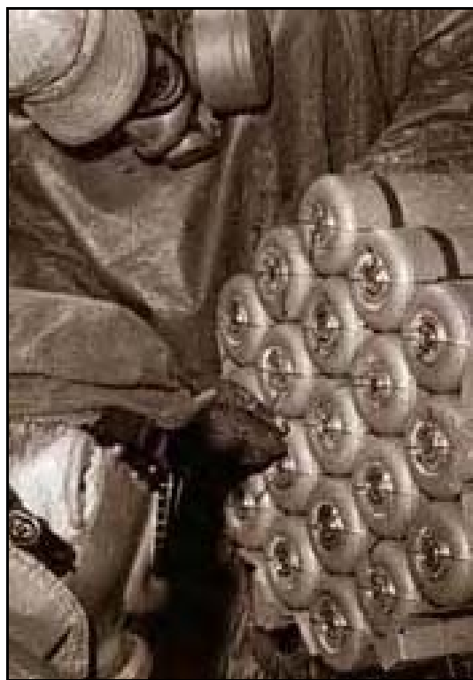
Figure 2.4. Technician deactivating fuses in cluster bombs at the Arsenal.
