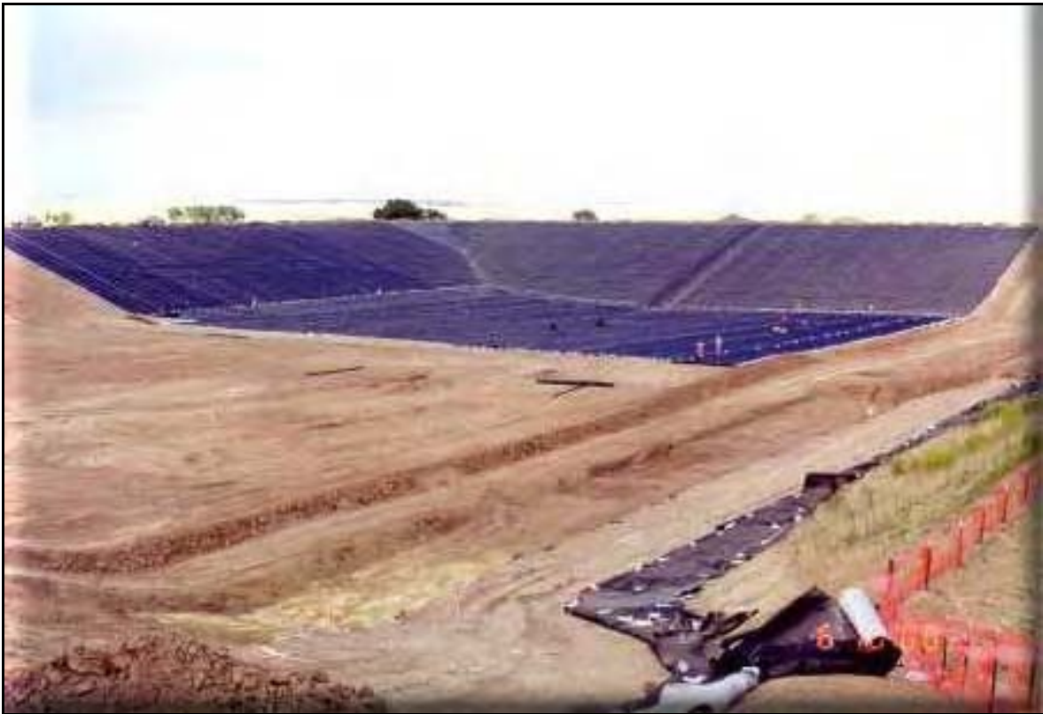
Figure 3.5. Construction of the lined on-post hazardous waste landfill for contaminated soils.
