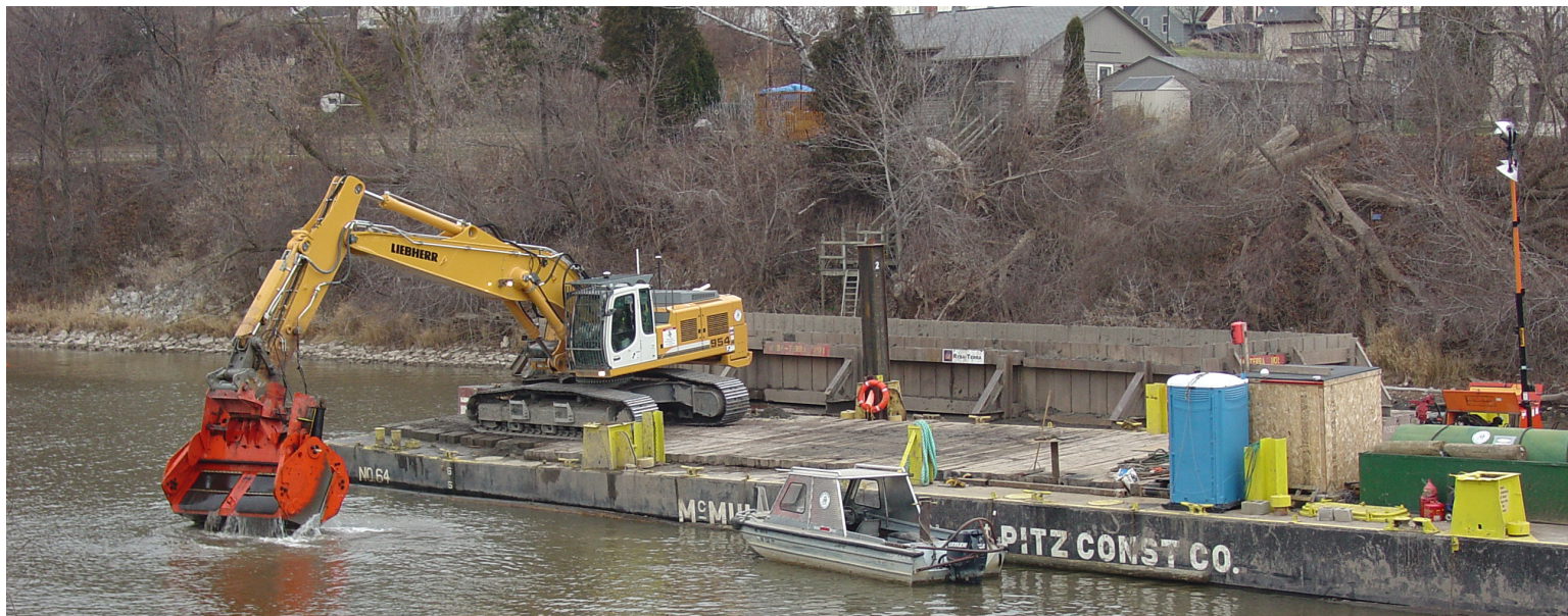
Excavating contaminated sediments from the Sheboygan River. Photo credit: Amy Kretlow.
