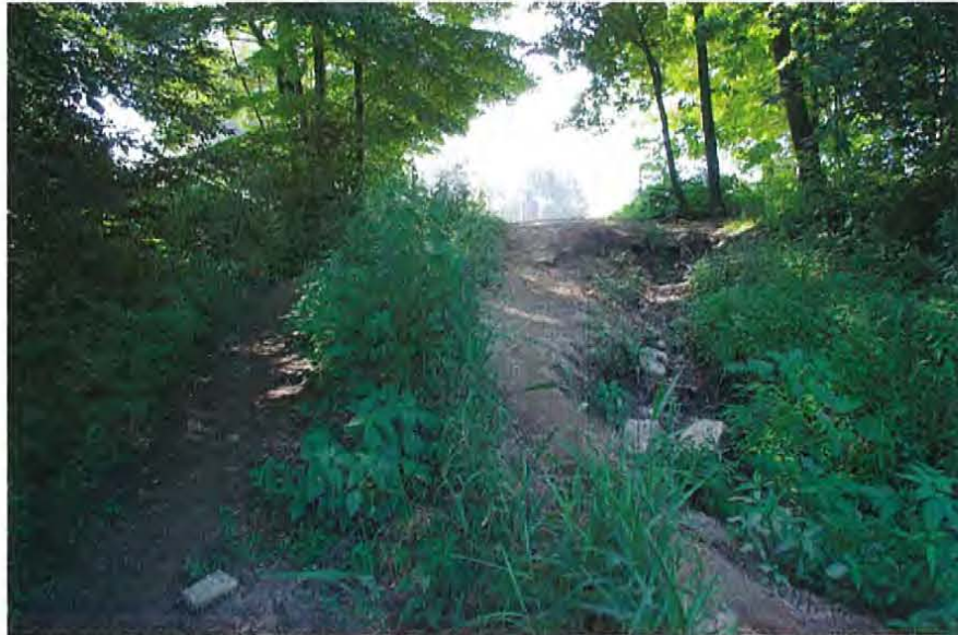
Figure 2. Erosion on boat launch path to Quinebaug River
