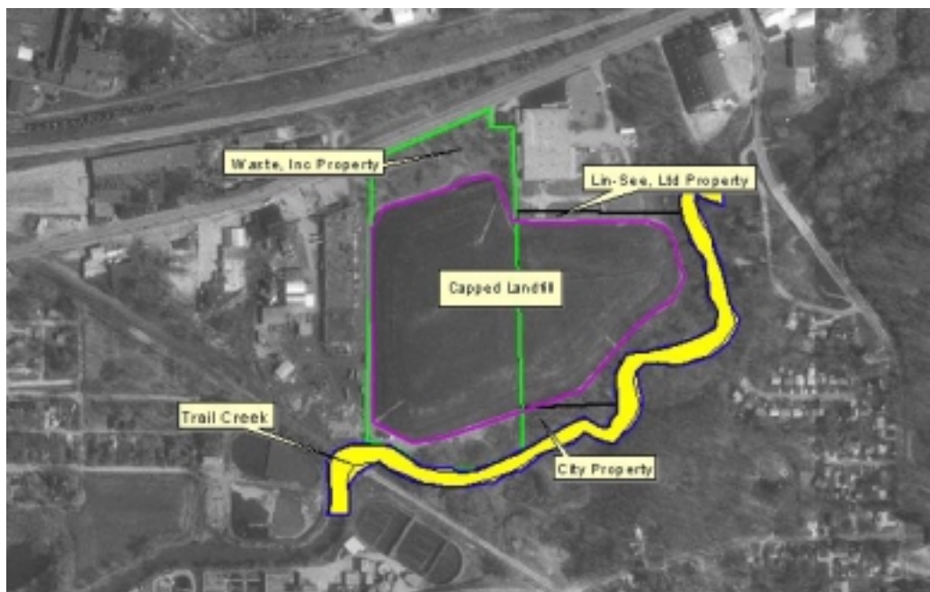
Figure 2. Waste, Inc. site following remediation. Original property boundaries included for reference only. (Photo source - US Department of Agriculture, Natural Resources Conservation Service, National Cartography and Geospatial Center, National Digital Orthophoto Program, Ft. Worth, Texas).
