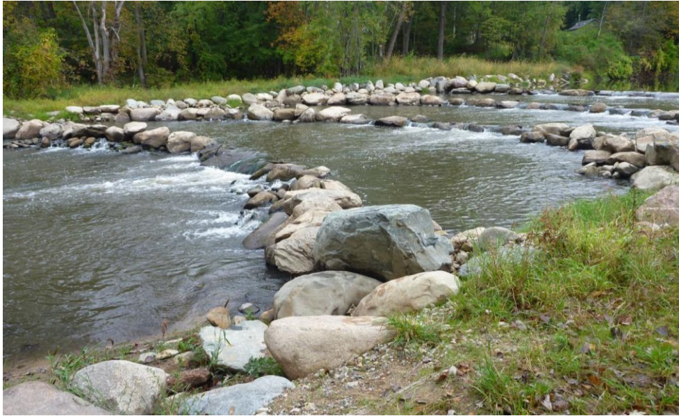
Figure 3.5. Rock ramp on the Thornapple River Village of Nashville, Michigan. This rock ramp replaced the Nashville Dam, which was removed in 2009, opening up 60 miles of stream to fish passage.
