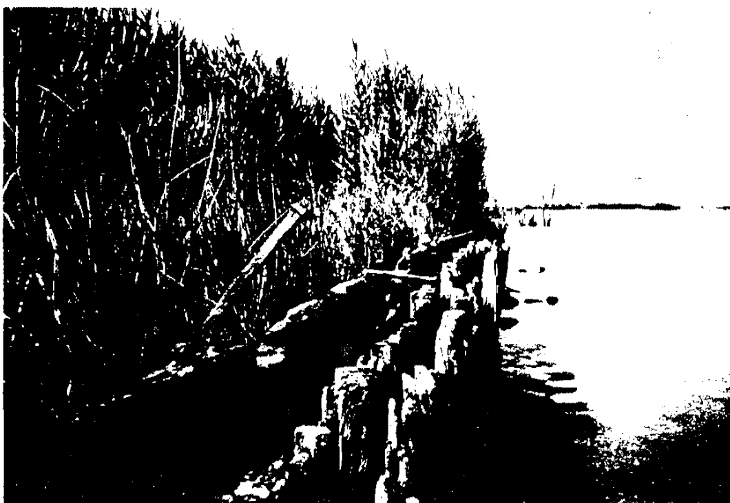
PHOTO 3: Outshore ("T") End of pier, from downriver, showing notched timber construction.
