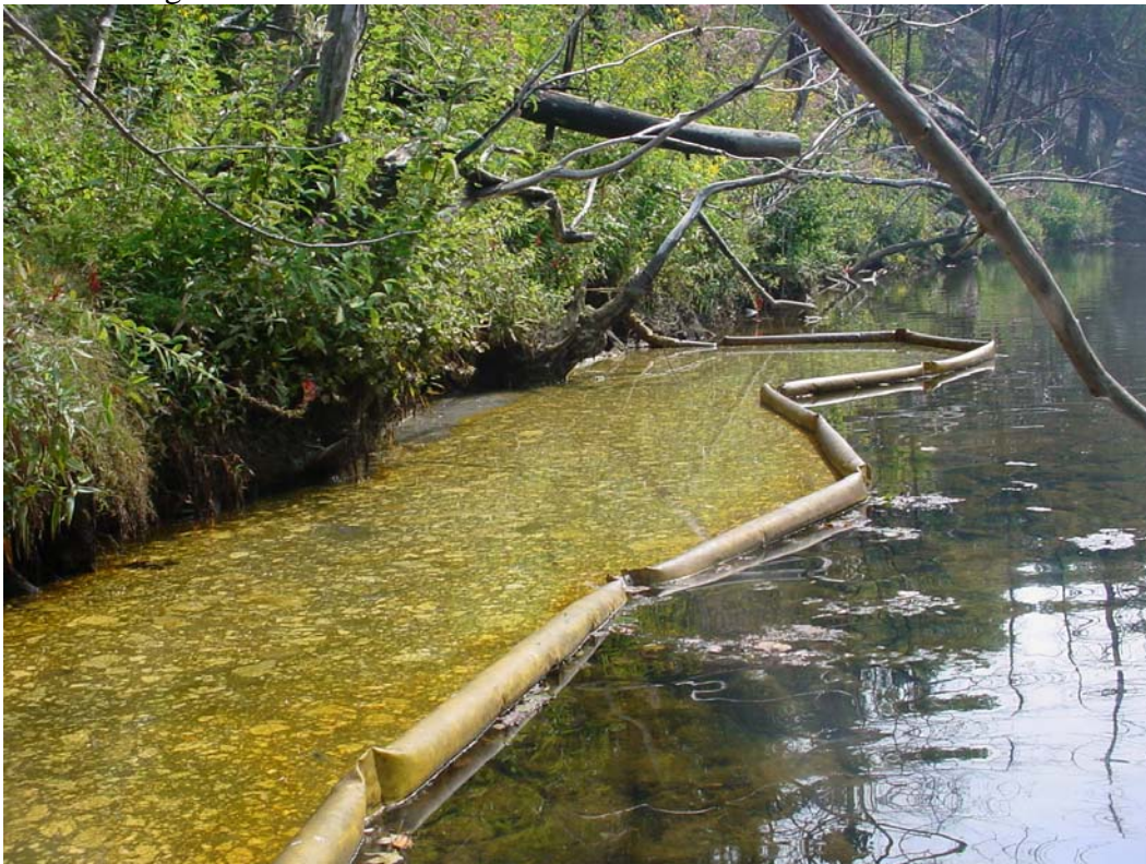
Figure 4. Oil accumulated within the boom at the spill site in Clear Creek. Photograph taken 17 August 2004.
