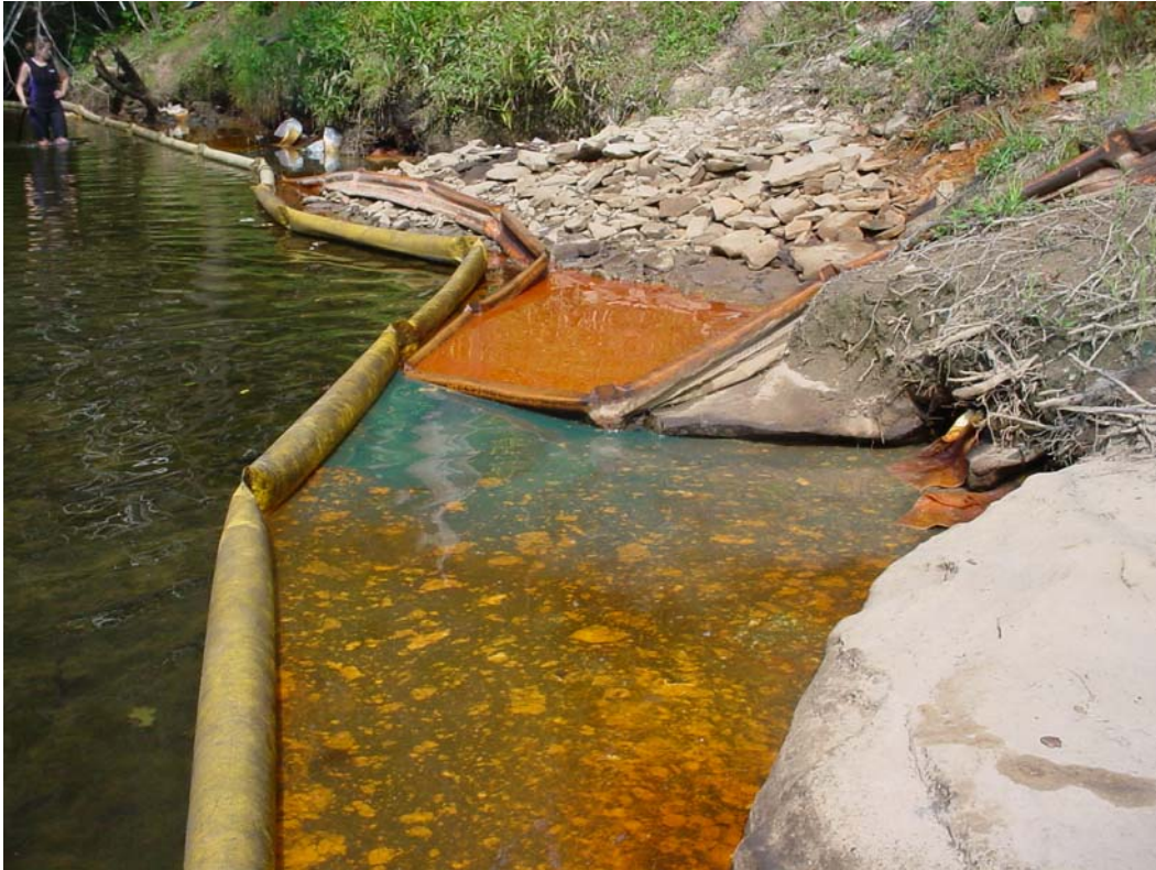
Figure 3. Oil accumulated within the boom at the spill site in Clear Creek. Photograph taken 17 August 2004.
