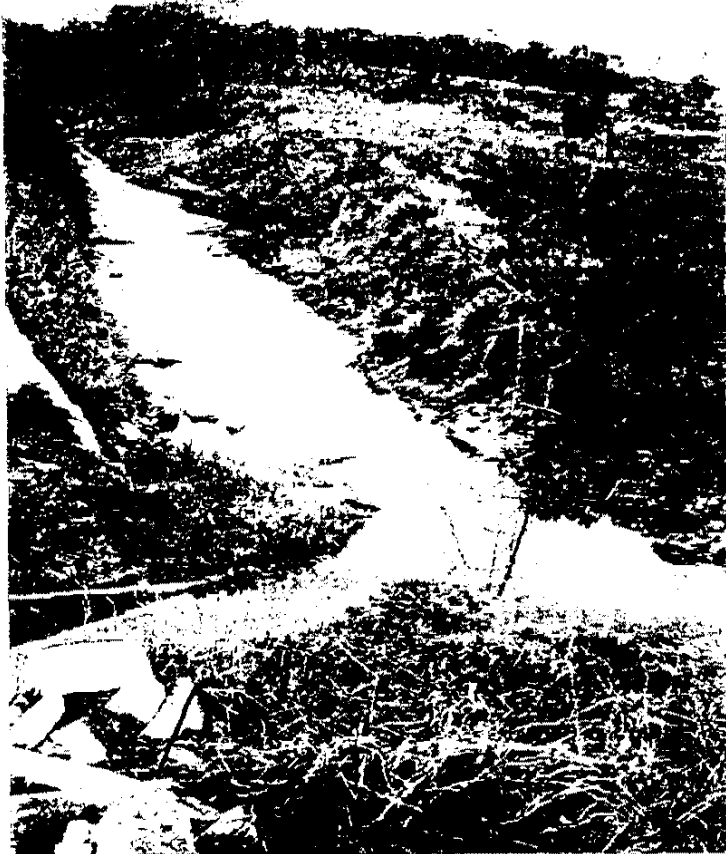
Secondary Infall Point: The ditch to center left is the Planned outfall from the southern half into the northern quarter. The ditch from top center will be extended outward into the adjacent higher land; in order to collect it's runoff for insertion into the new water treatment system.
