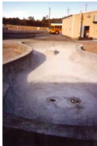
A demonstration pond was constructed at Junction School.
