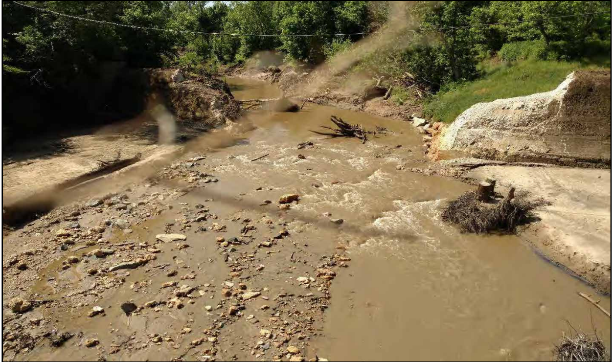
29. Cobble and gravel sediment transport through breach in dam (5/25/17)
