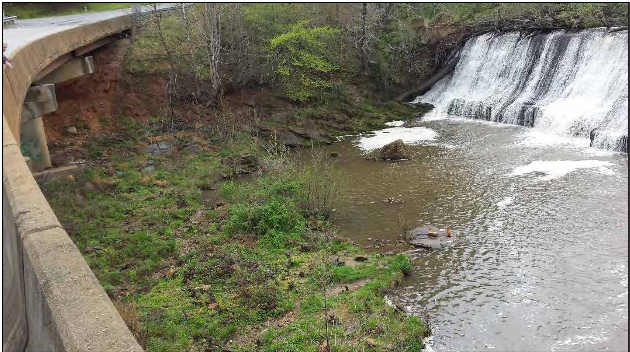
6. Over-widened channel and scour hole on right bank below Power Dam, view east (4/16/15)
