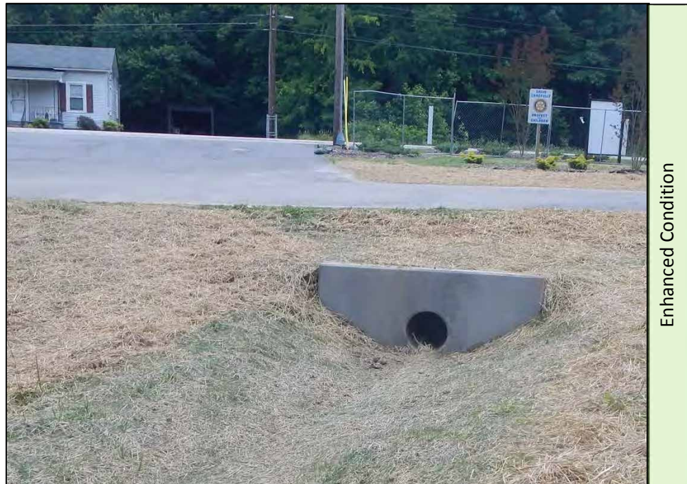
Picture 8: New headwall added to existing culvert.
