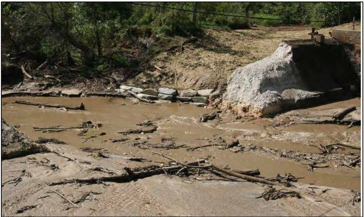
24. View of left bank upstream of dam after stacked stone toe, backfilling, and matting stabilization (10/5/16)
