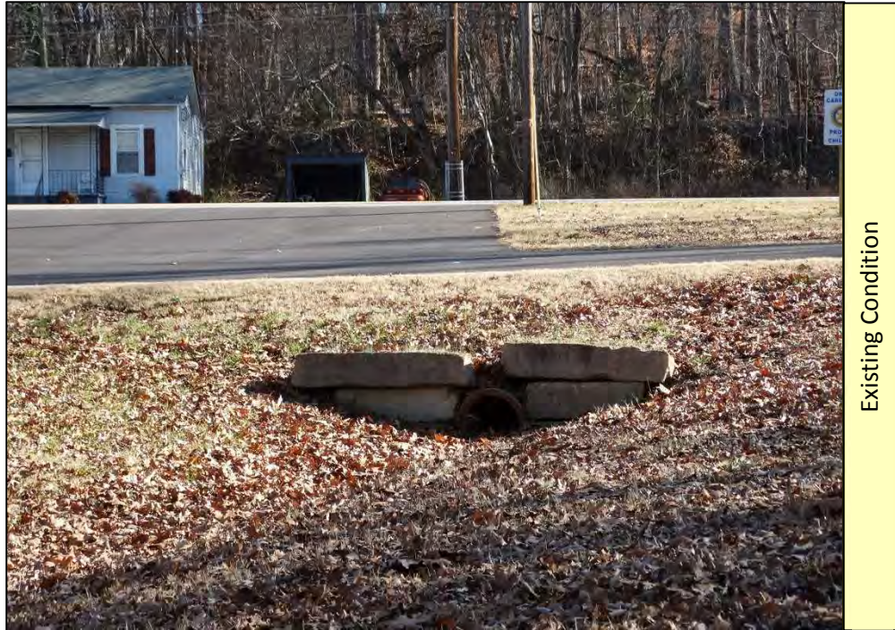
Picture 7: Existing culvert to receive new headwall.
