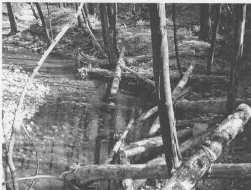
Figure 29: Completed placement of woody debris in stream
