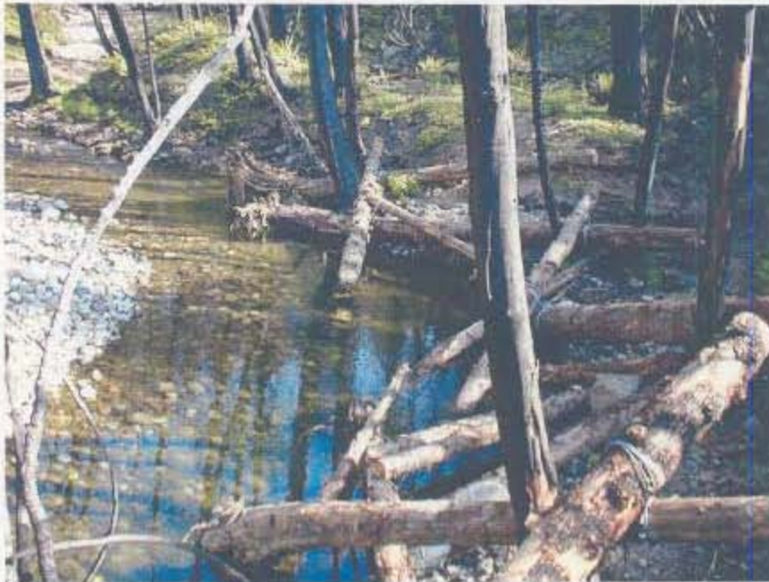
Figure 29: Completed placement of woody debris in stream
