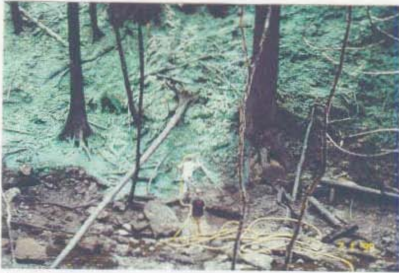
Figure 23: Hydroseeding
