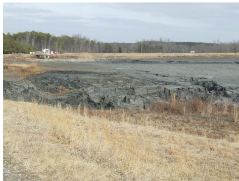
USFWS, A pipe rupture caused the coal ash slurry impoundment to drain into the river.
