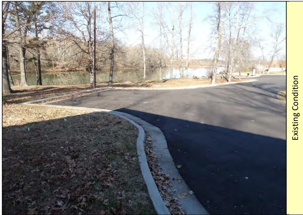
Picture 21: Existing parking spaces. Portion of curb to be removed to create accessible parking for future sidewalk to connect to the restroom and fishing platform.
