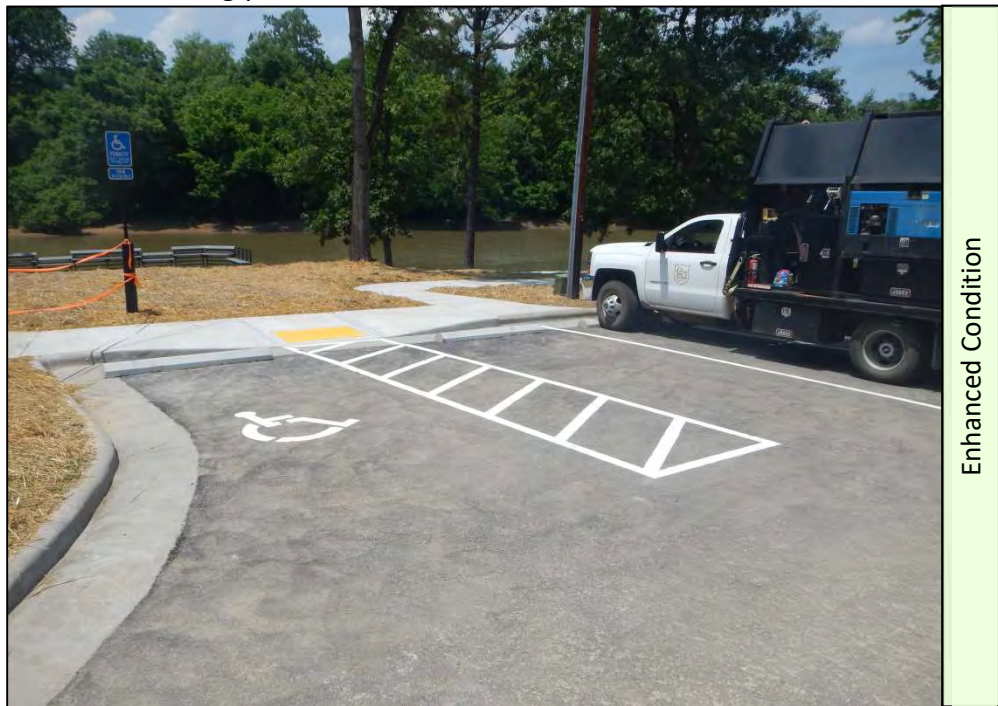
Picture 22: New accessible parking spaces with accessible sidewalk connecting to the restroom and fishing platform.
