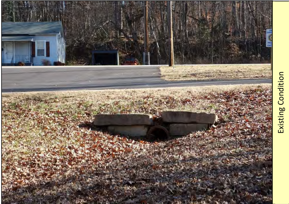
Picture 7: Existing culvert to receive new headwall.
