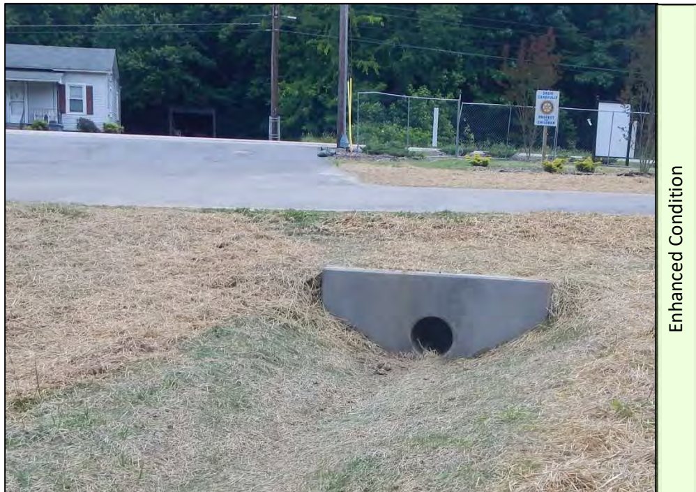
Picture 8: New headwall added to existing culvert.
