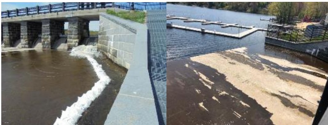
Figure 18. Mystic Lake Dam and Shallow Flow onto Spillway (right image) and Sandbags Used as a Temporary Solution to Promote Fish Passage (left image)
