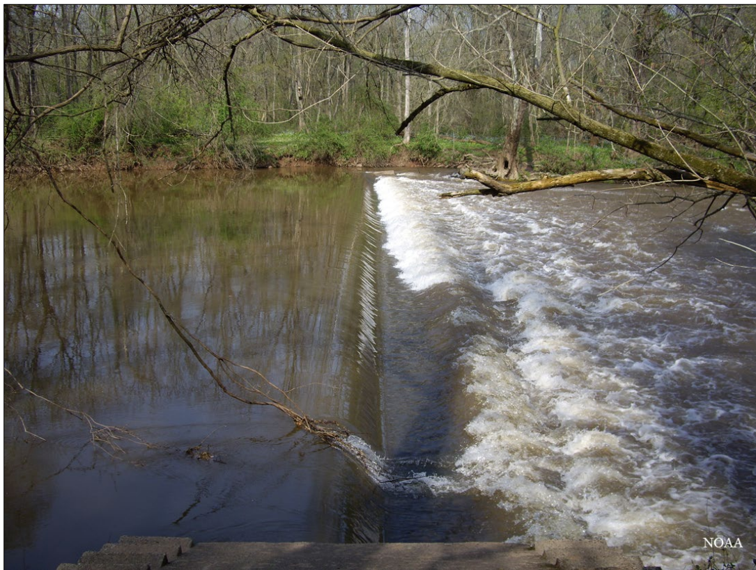
Figure 19. Mill Lane Dam shown facing northeast. Water has eroded the stream bank along the northeastern edge of the dam, and visibly flows around the weir.
