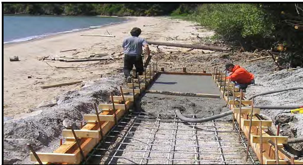
ADA ramp construction at Quarry Beach.
