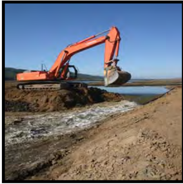
Excavator removes final portion of levee, allowing creekwaters to flow into the Giacomini Ranch's East Pasture.
