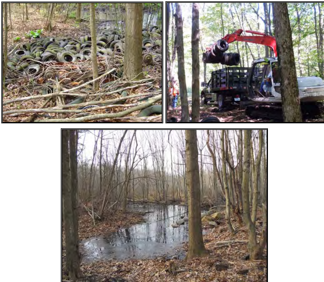
Figure 4. Tire dump in forested wetland before, during, and after tires were removed.
