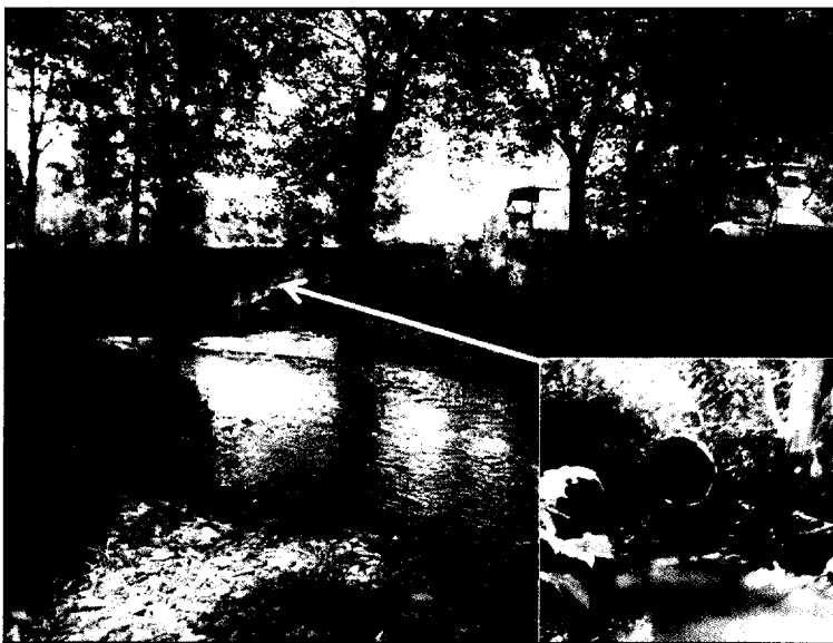
Figure 3. Corrugated plastic pipe storm drain outlet.
