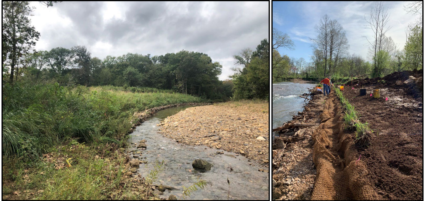
Streambank restoration photos depicting restoration elements proposed for the Sycamore Creek streambank stabilization project. Images shown include post-restoration condition of stream reach in Arkansas showing riffle, pool, and grade control using toe-wood and construction of vegetated flood plains (left panel); and construction and planting of soil lifts on toe-wood structure (right panel).
