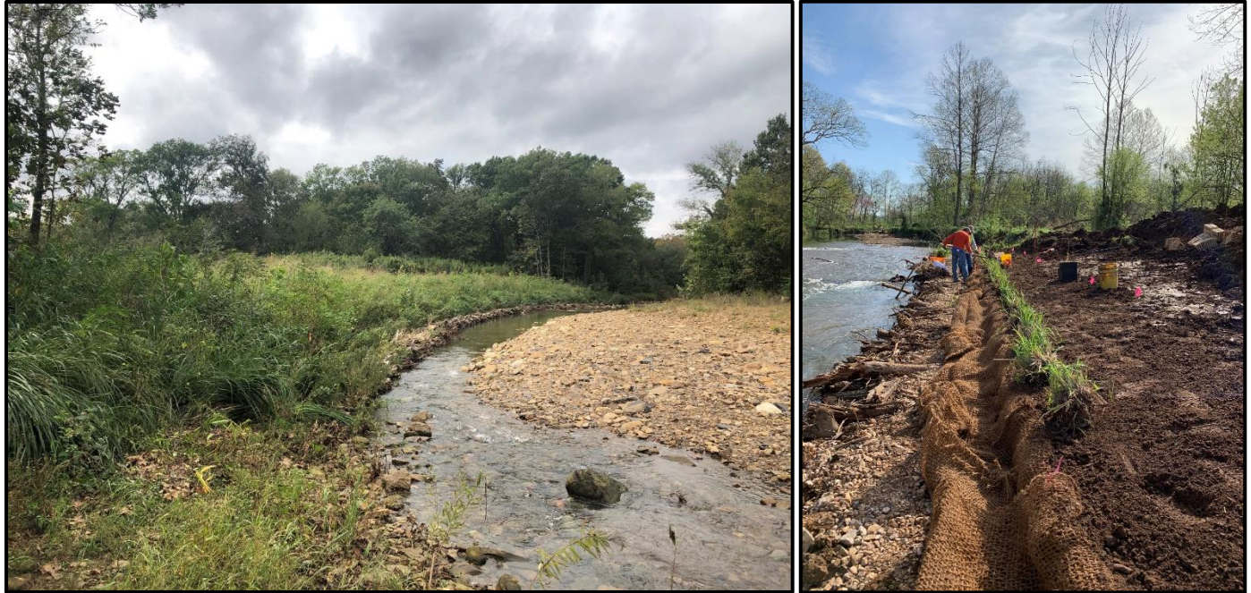
Figure 6. Streambank restoration photos depicting restoration elements proposed for the Sycamore Creek streambank stabilization project. Images shown include: post-restoration condition of stream reach in Arkansas showing riffle, pool, and grade control using toe-wood and construction of vegetated flood plains (left panel); and construction and planting of soil lifts on toe-wood structure (right panel).
