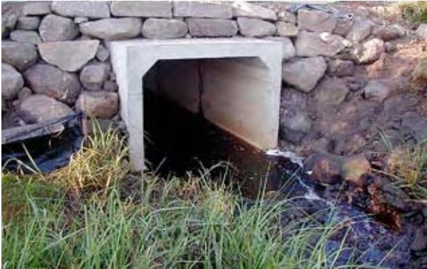
Figure 4.4. Example of a simple open box culvert (Massachusetts Department of Fish and Game, 2005)
