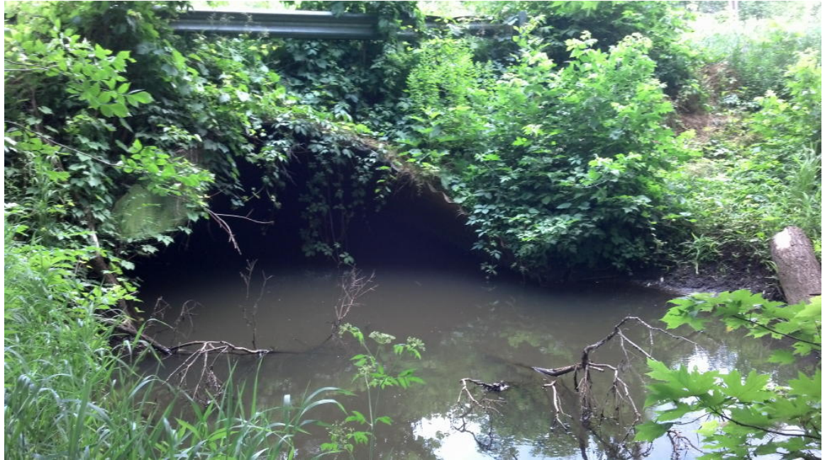
Figure 4.6. Flooding at 30 Mile Road because of flow being impounded at 29 Mile Road crossing (Calhoun County Conservation District)
