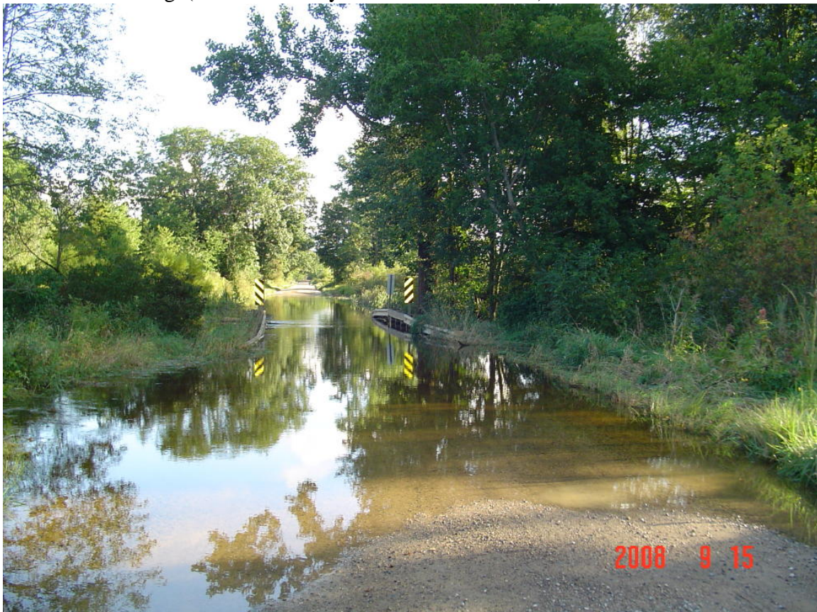
Figure 4.6. Flooding at 30 Mile Road because of flow being impounded at 29 Mile Road crossing (Calhoun County Conservation District)
