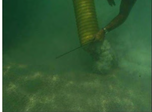
Fill Being Deposited in Blowhole
