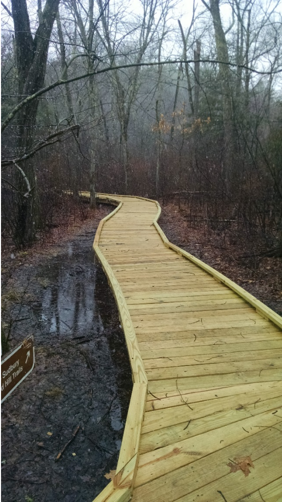
Photos 5 and 6: Boardwalk over wettest sections of trail
