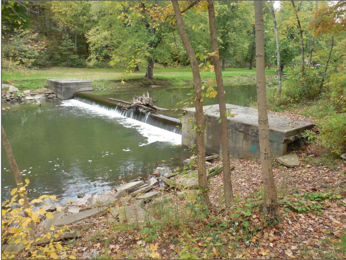
Figure 14. View of dam from east bank showing weir and abutments, view looking northwest
