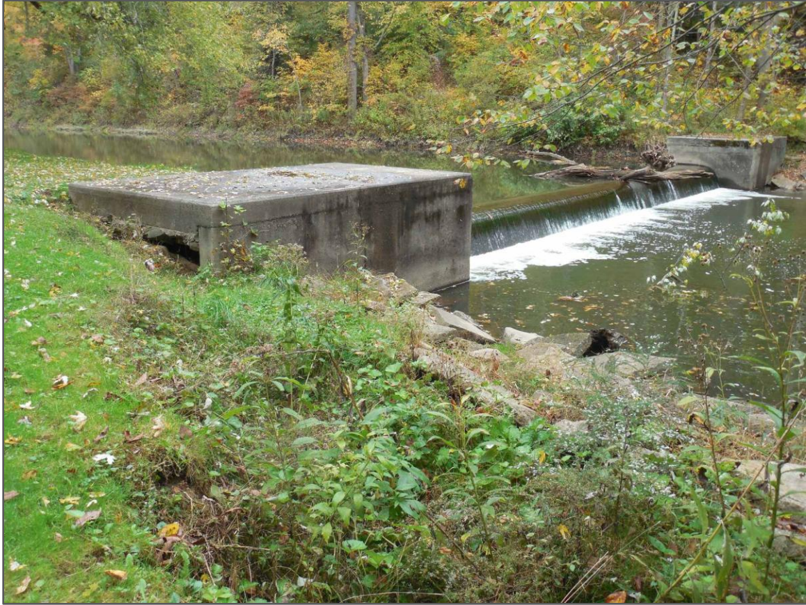
Figure 15. West abutment showing void and erosion, view looking northeast
