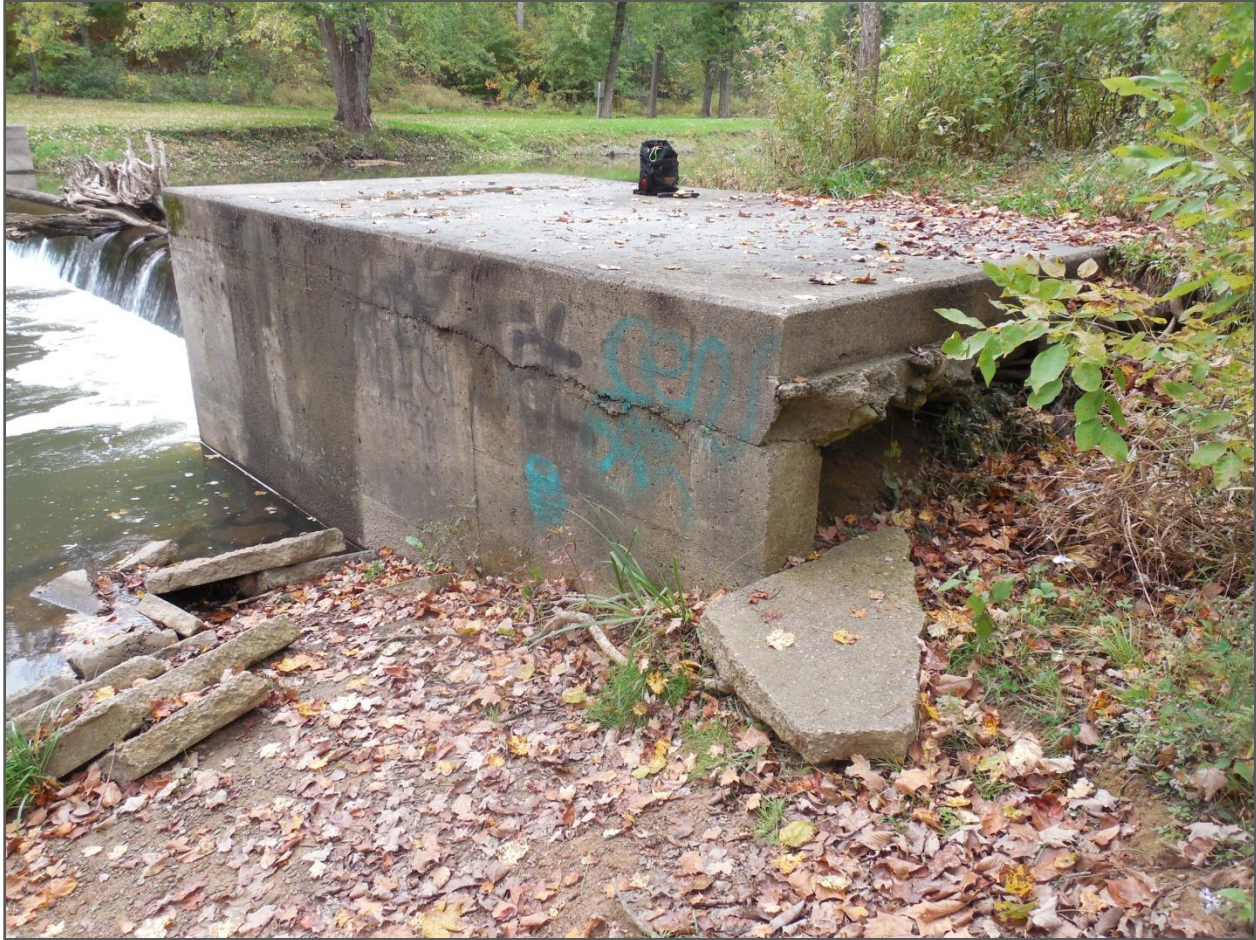
Figure 16. East abutment showing irregularly poured top slab, view looking northwest
